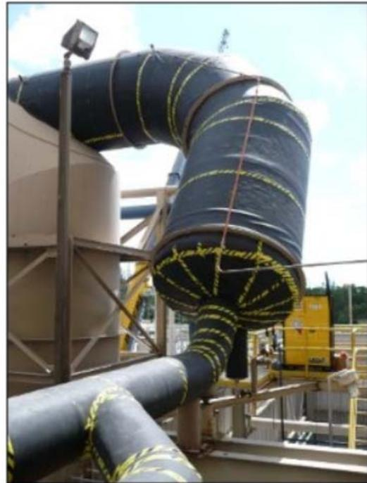
**Industrial noise pollution solution:** before and after application of Acoustiblok, sound reading registered an amazing 26-28 dB attenuation, which translates to a human ear perceived noise reduction of 90-percent.
